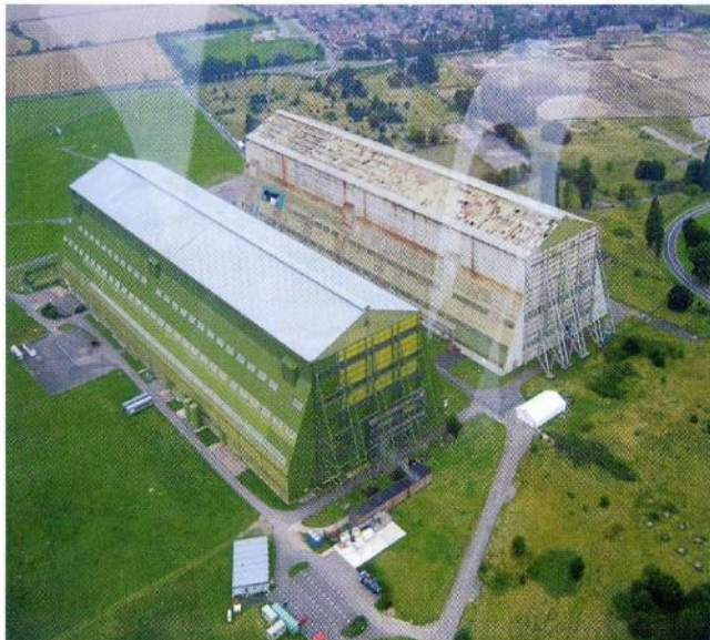
▲ The twin sheds at Cardington still stand as gigantic monuments to the Imperial Airship Scheme to link the empire. Photographed from the Zeppelin NT07 003 in August 2008.
